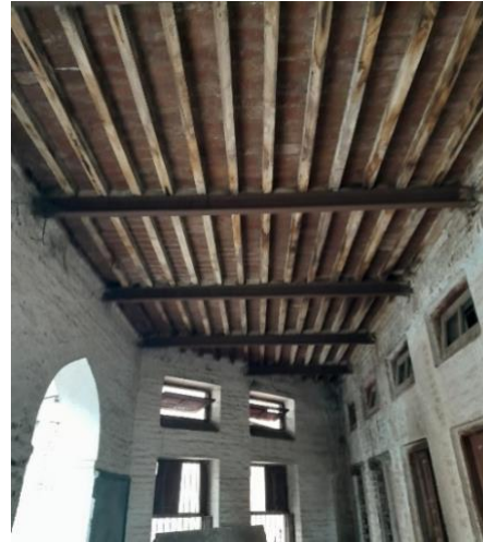
Figure 15: inside view of the building with Wood Roof (Author 2024)
