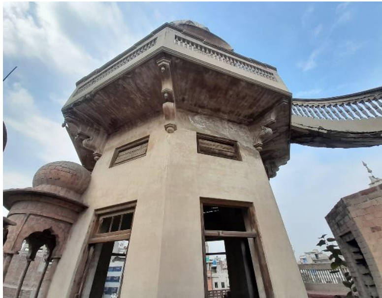
Figure 20: Domes structures on the top of the building (Author 2024)
