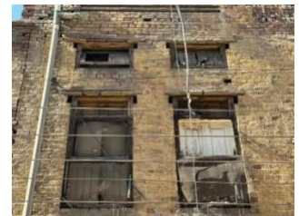
Figure 11: Brick work and Wood work on the Facade
