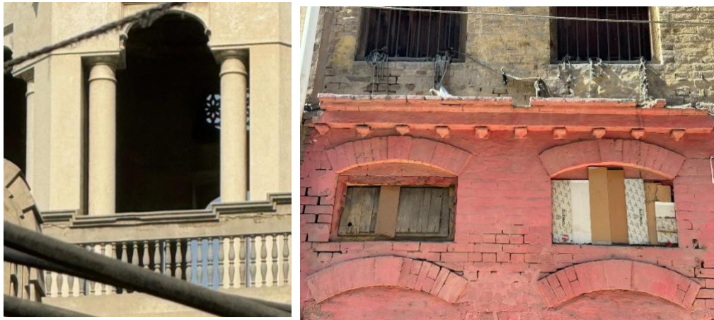
Figure 19: Semi circular arches on the top of Windows on the Building Facade (Author 2024)
