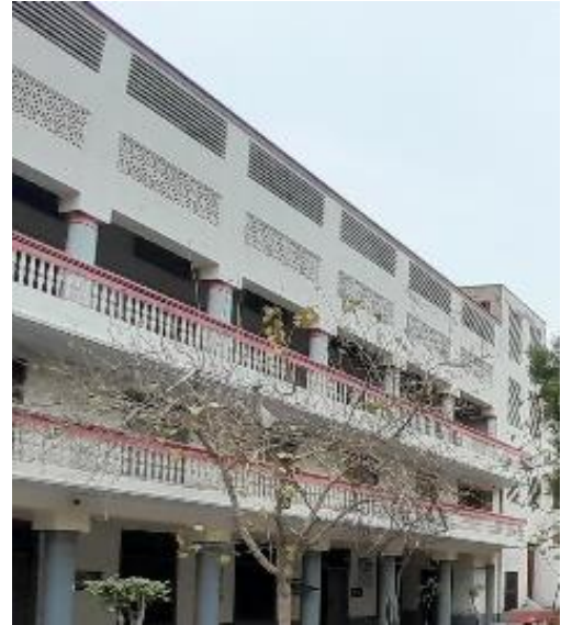
Figure 18:jali Work on Every Floor of the building (Author 2024)
