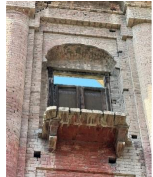
Figure 10: brick work and arches with cantilevered features (Author 2024)
