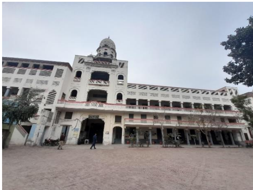
Figure 12: inside elevation of the building block from the central courtyard (Author 2024)
