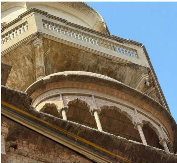
Figure 24: jharoka, terracotta jali, arches and columns on top of the building (Author 2024)
