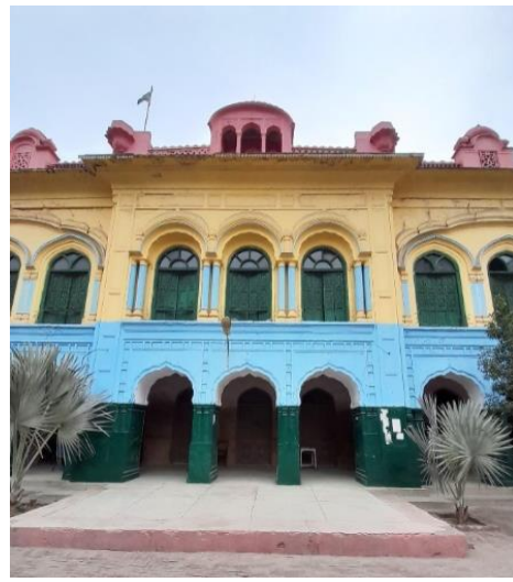
Figure 14:north-West side elevation from the central courtyard (author 2024)
