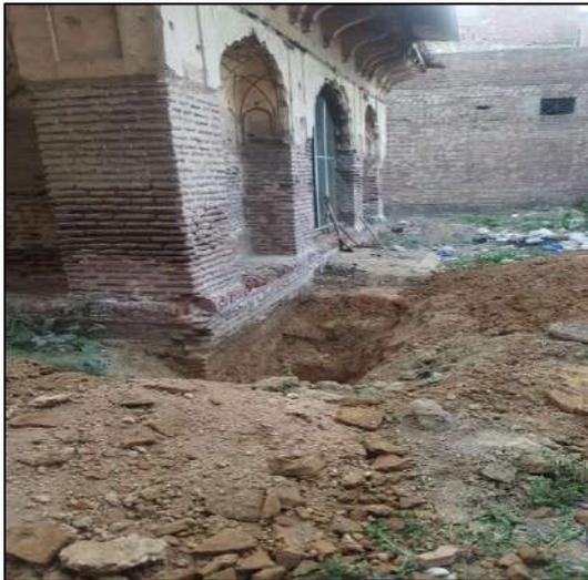
Figure 17 digging for foundation
