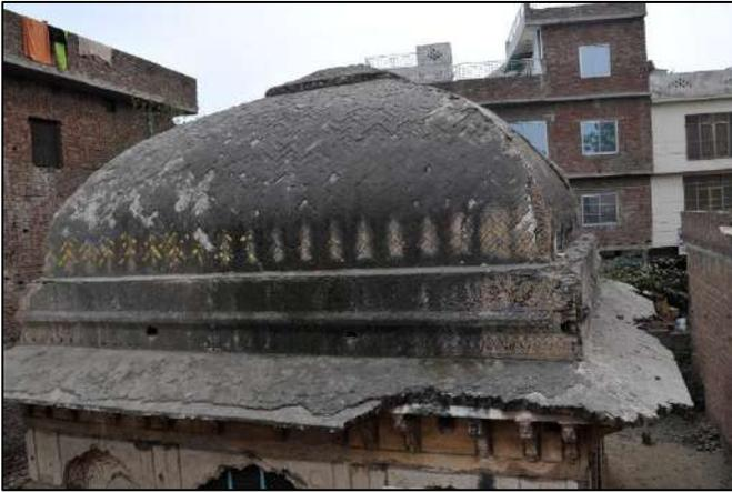
Figure 18 Exposed Brick Brackets (highlighted)
