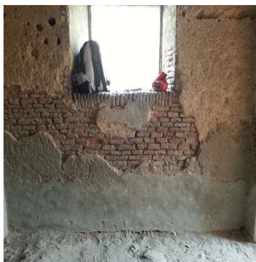
Figure 10: Damaged Plaster, Cracks in building, damaged brick masonry and decayed wood (Source: WCLA)
