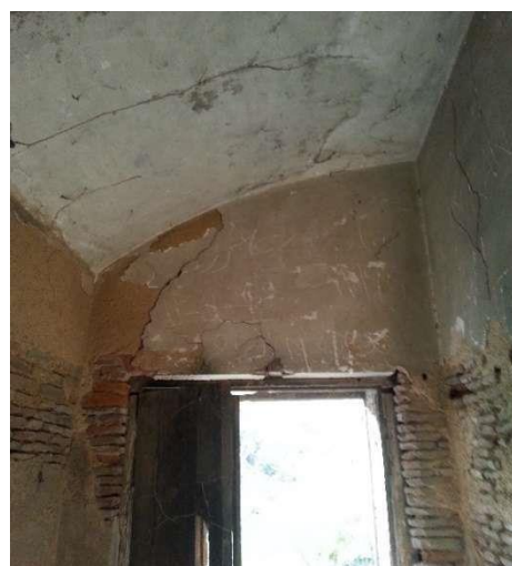
Figure 10: Damaged Plaster, Cracks in building, damaged brick masonry and decayed wood (Source: WCLA)
