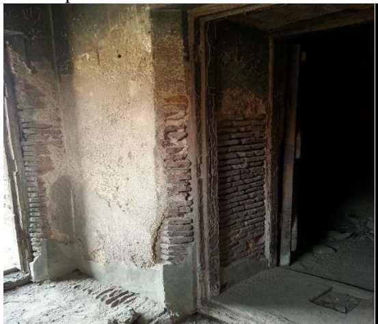
Figure 12: Image showing structural damages such as peeling of lime pilaster and rotten bricks (Source: WCLA)
