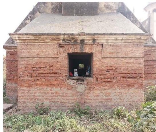
Figure 12: Image showing structural damages such as peeling of lime pilaster and rotten bricks (Source: WCLA)
