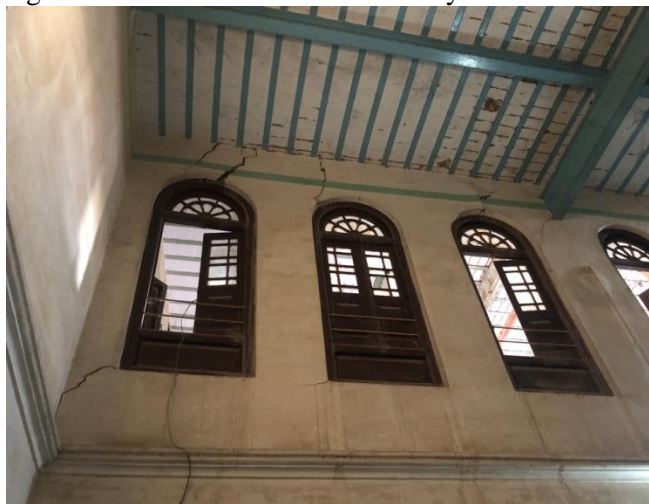
Figure6: shows the roof built by I beam, T iron and burn bricks. (a house built in 1930 at Awan Muhala)
