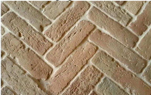
Figure11: backed brick floor
