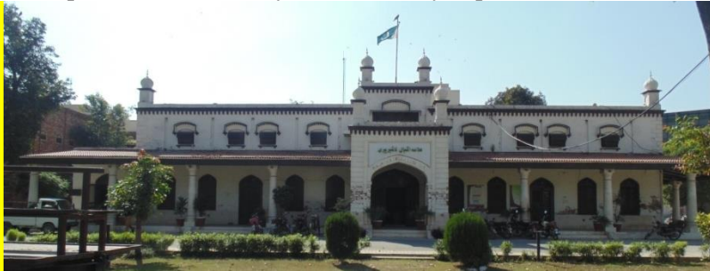
Figure-8: Façade of the building (Source: Author)
